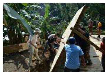
Raising new bathroom wall
