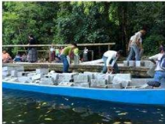
Concrete blocks at the dock
