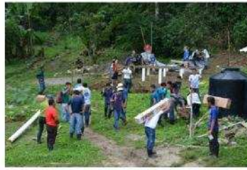
Building the foundation
