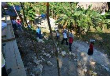
Moving concrete blocks
