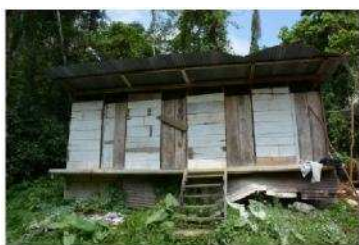
Former bathrooms (pew)
