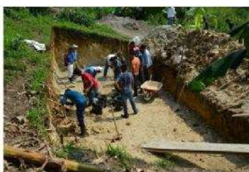
Digging out new bathroom site
