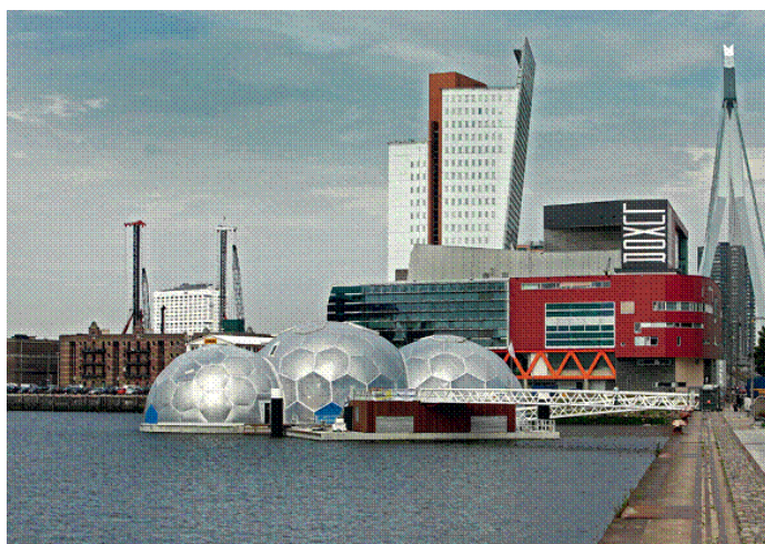
Figure 4.5: Floating Pavilion in Rotterdam the perfect show case of adaptive building
