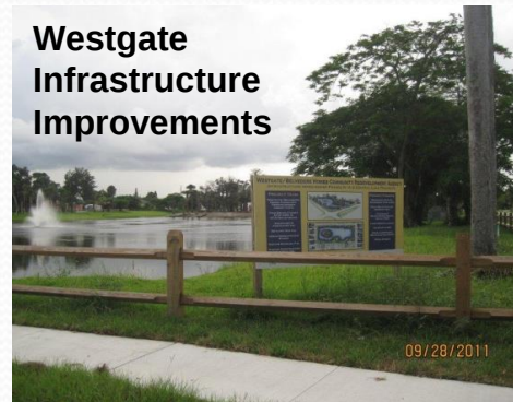
West Palm Beach Stormwater Improvements
